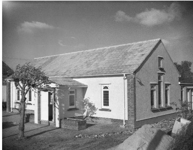
Photo of the Church in November 1954 just prior to re-opening
