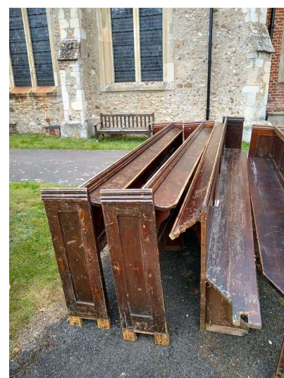
Removal & Replacement of the pews
