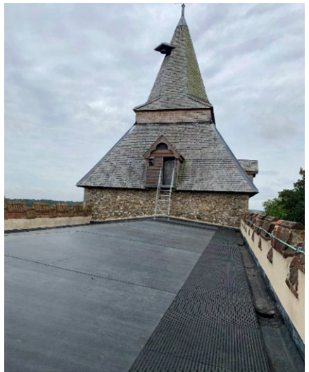
New Nave Roof
