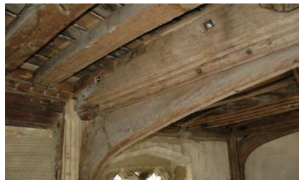
New Flitch Plate Installed in Ridge Beam
