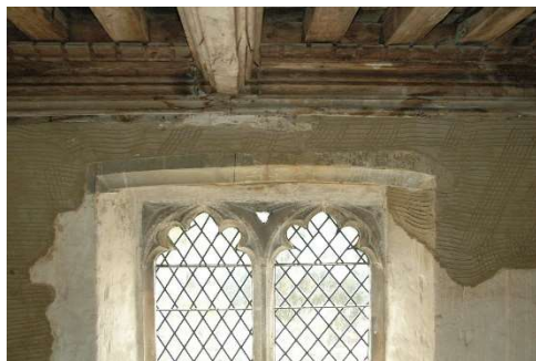
Repairs to Clerestory Window
