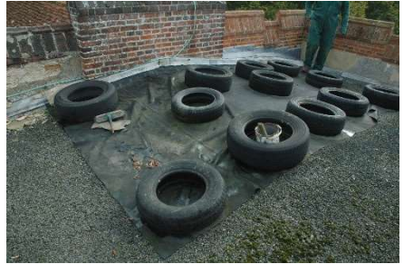
Roof Pre Repairs
